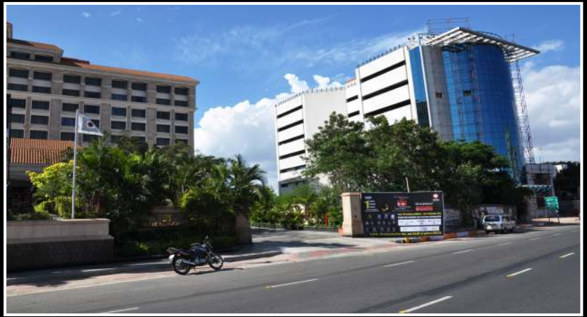
Hoarding at the Entrance of The Hotel Residency
